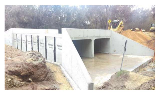
The size of the culvert in the picture is higher than would be needed, but Pallinup South would need an extra barrel (using link slabs) making it lower but wider. Councillor Dennis inspected the culvert on our way to the RRG meeting in Woodanilling to get an idea of the size and cost.
